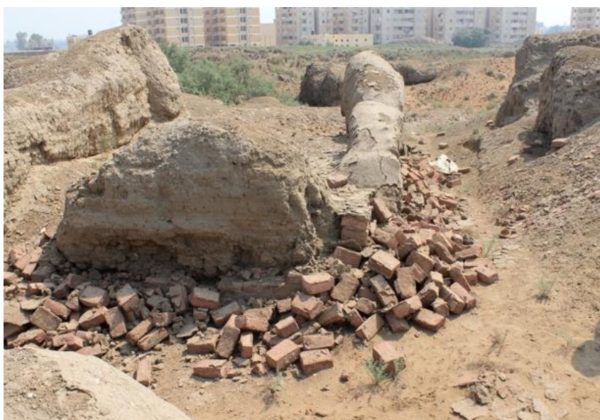
Figure 12. The destroyed 2013 restoration in Unit Q13-1.
