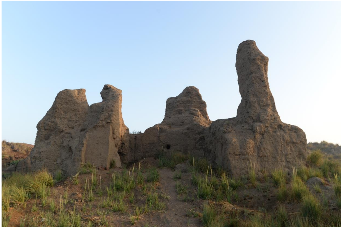
Figure 14. Unit L14 after conservation.
