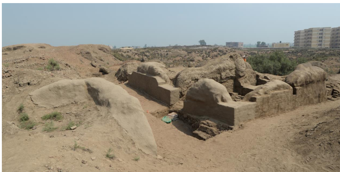
Figure 13. Unit Q13-1 after repair and conservation of the damage.
