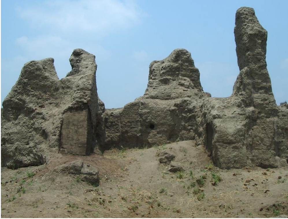
L14, Building #1, After Intervention.
