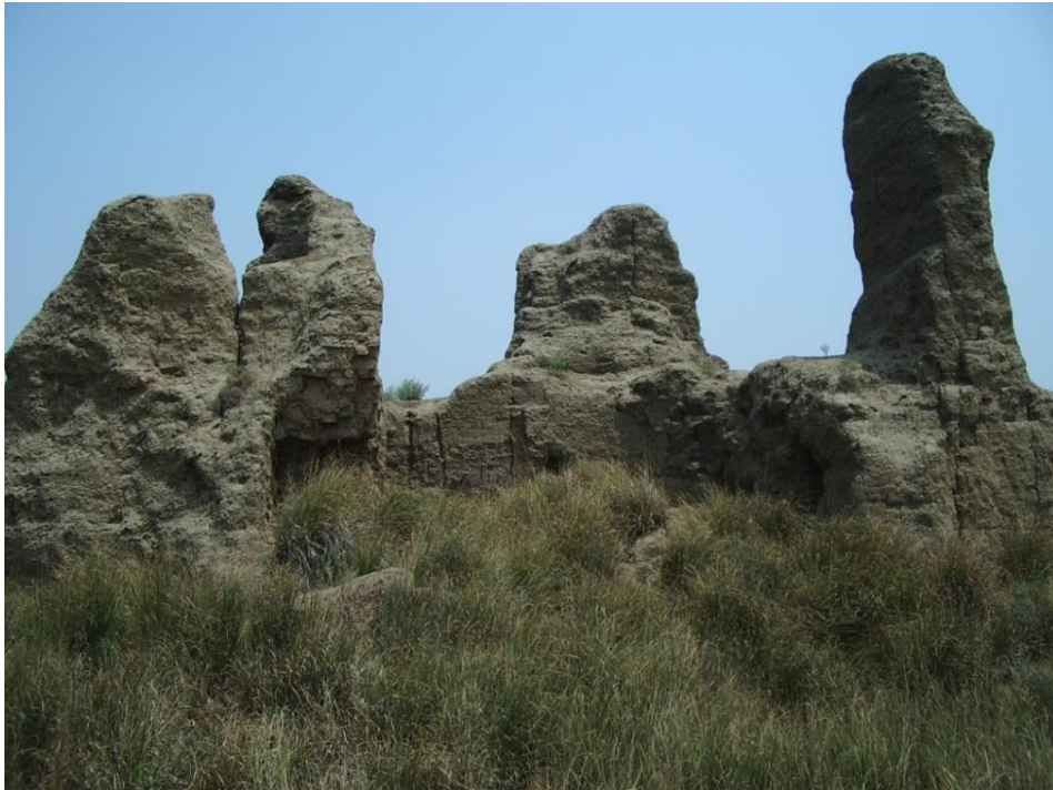
L14, Building #1, Before Intervention.
