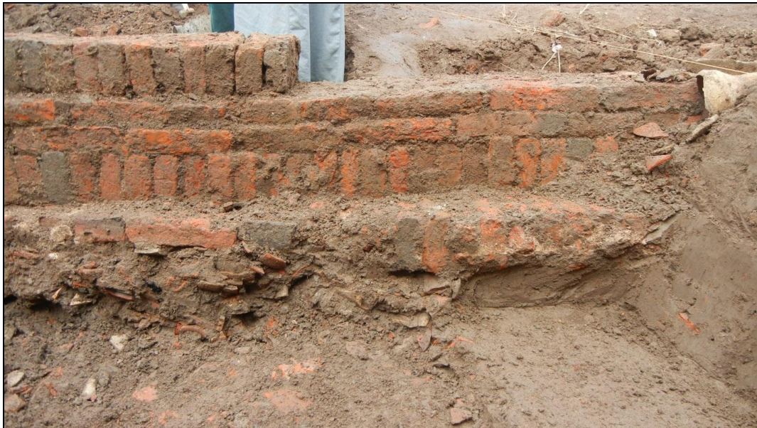
Figure 3. Coursings of the brick wall (view west).
